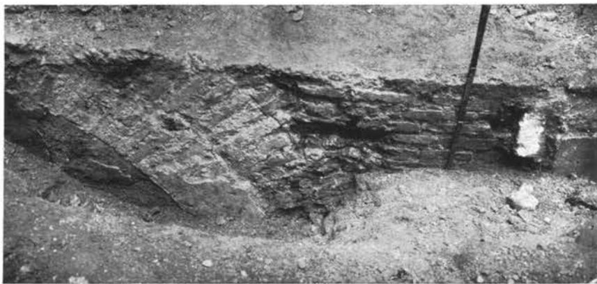
Fig. 126 — S. Lorenzo in Damaso. Brick wall with secondary arches found in the palace courtyard (Photo: Sansaini)
